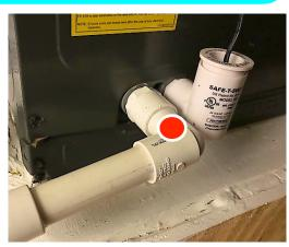
Locate the A/C drain coming out of the handler and drill a 5/32" (4 mm) hole through the TOP of the pipe (or fitting) close to the A/C handler as shown by the red spots.
