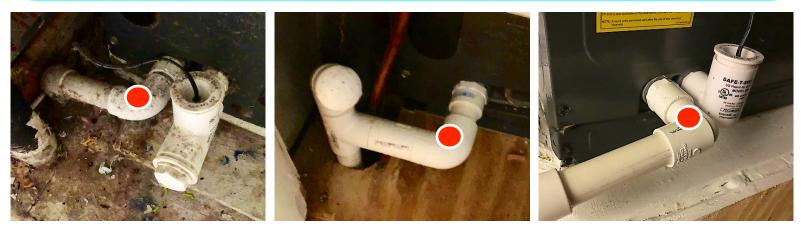
Locate the A/C condensate drain coming out of the handler. Drill a 5/32" (4 mm) hole through the TOP of the pipe (or fitting) close to the air handler, but away from a panel, as shown by the red spots.
